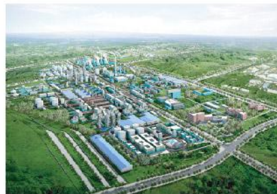
新疆中泰电厂/闭式水冷却器/AN40L3 Xinjiang Zhongtai electricity generating station
