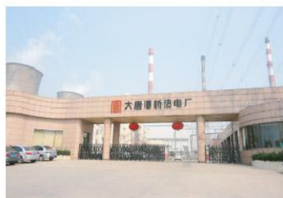
西安灞桥电厂/闭式水集装装置 Xi'an Ba Qiao electricity generating station
