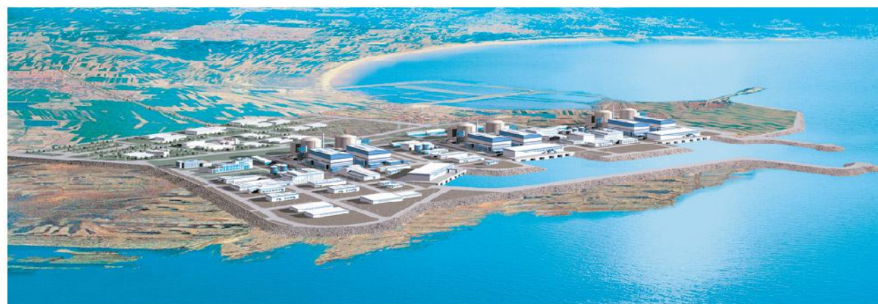
山东烟台海阳核电 Shandong Yantai Haiyang Nuclear Power Plant
